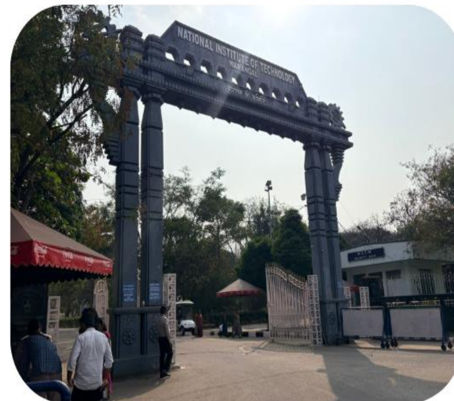
Renovation of Main Gate
